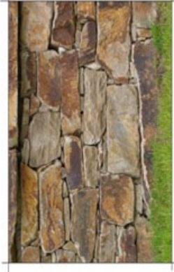
RETAINING WALL: NATURAL 'DRYSTONE' GARDEN WALL
