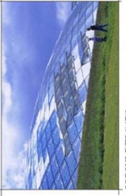
DOPE ROOF: TINTED GLAZING
