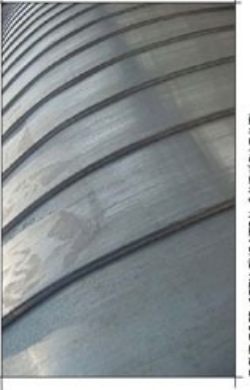
DOPE ROOF: GREY ZINC METAL SANDWICH PANEL
